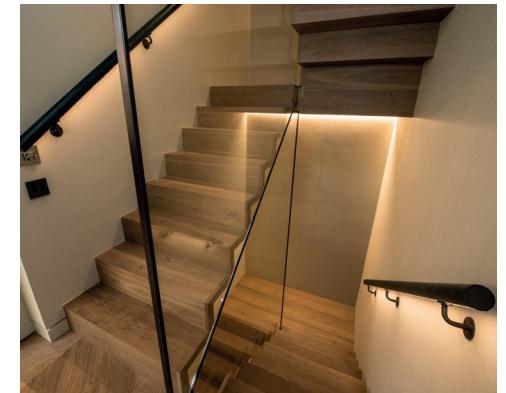
LED lighting under handrails and in stairwells.
